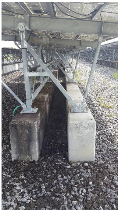
Figure 6: Mounting Structure Supporting PV Panels
