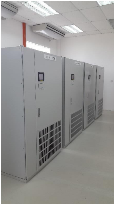
Figure 7: Left - Power Conditioning Systems (PCSs); Right - A PCS displaying the AC power output over one week period
