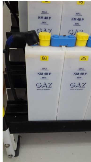
Figure 8: Nickel-Cadmium Battery Bank System
