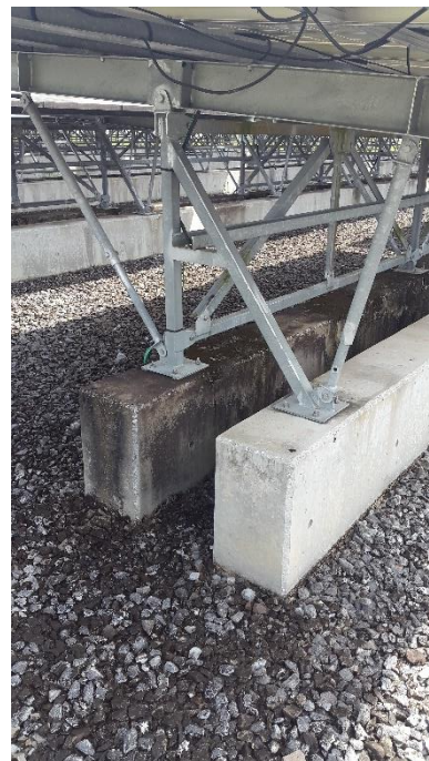
Figure 6: Mounting Structure Supporting PV Panels
