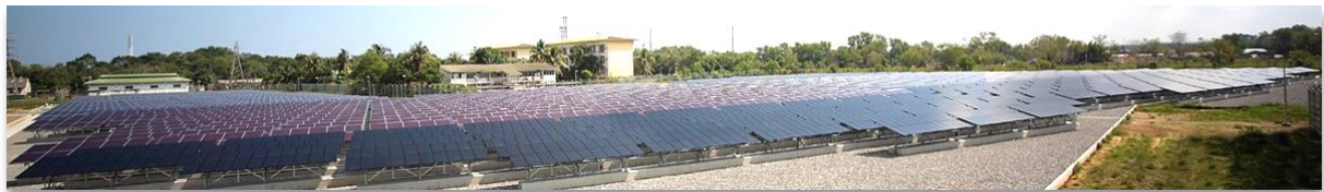
Figure 2: Completion of Tenaga Suria Brunei
