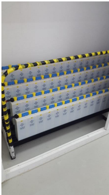
Figure 8: Nickel-Cadmium Battery Bank System
