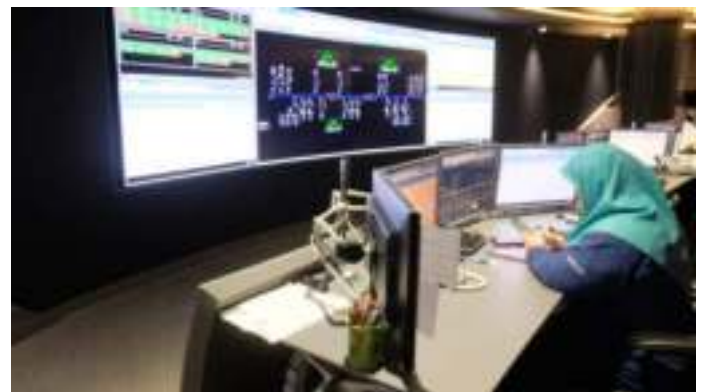
Supervisory Control and Data Acquisition (SCADA)
